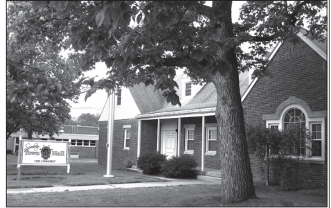
Speedway Town Hall, built in 1926, was the first location of the police and fire departments.
